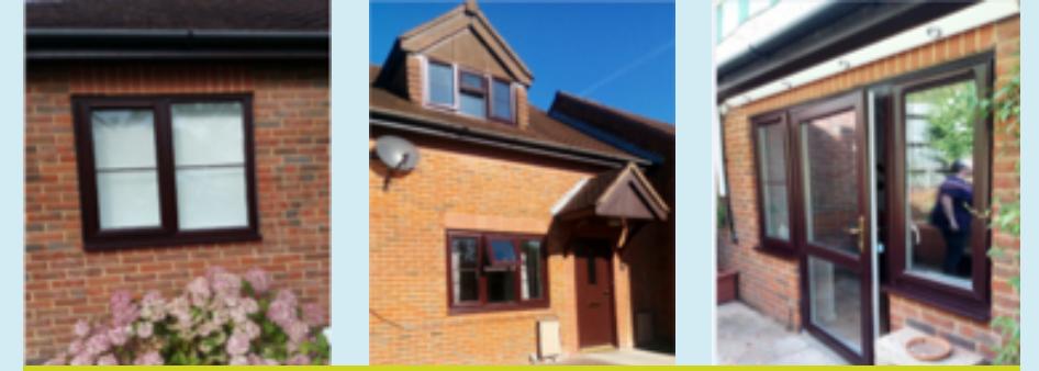
New windows and doors at Balfour Estate
